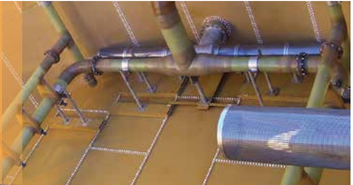
IFAS (Integrated Fixed-Film Activated Sludge)
